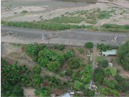
The fault surface rupture sheared a levee.
