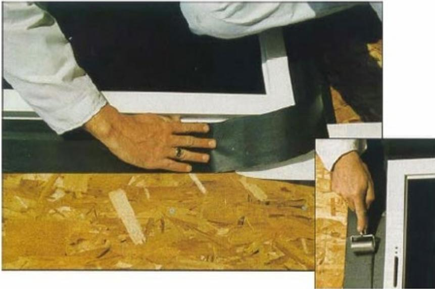
Example of self-adhering waterproof underlayment used to tape plywood joints, ridges and eaves. Photo depicts use around fenestrations.
