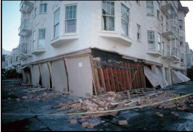
**Ground levels are no longer visible because of structural failure and sinking due to liquefaction. San Francisco, Loma Prieta, 1989 (USGS)**
