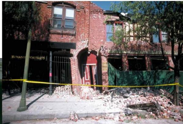
**Structure moving off an unsecured foundation**
